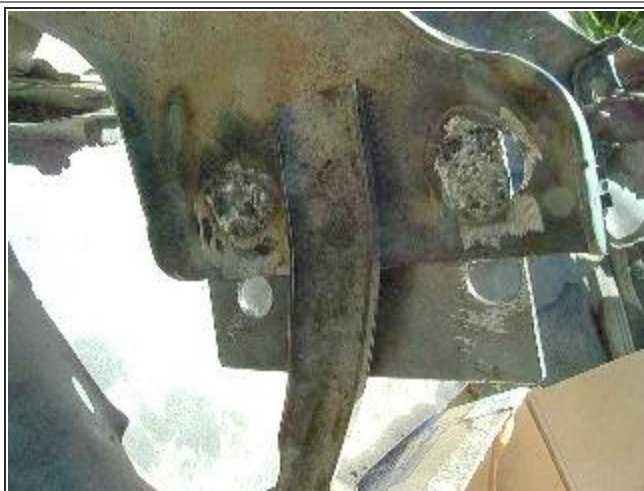
Bumper bracket optionally welded in place
