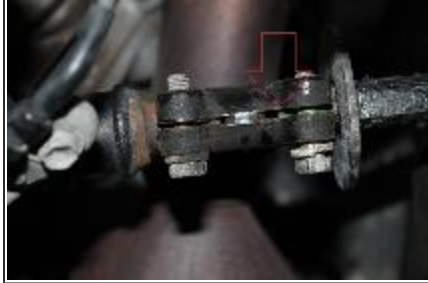
Steering Shaft Slip Joint - typical
